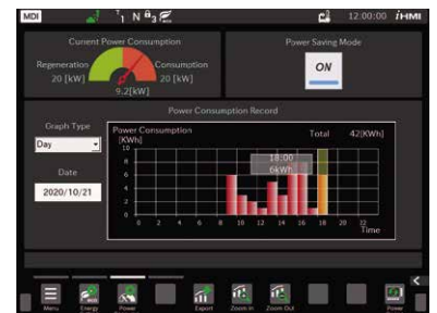
Power consumption monitor
